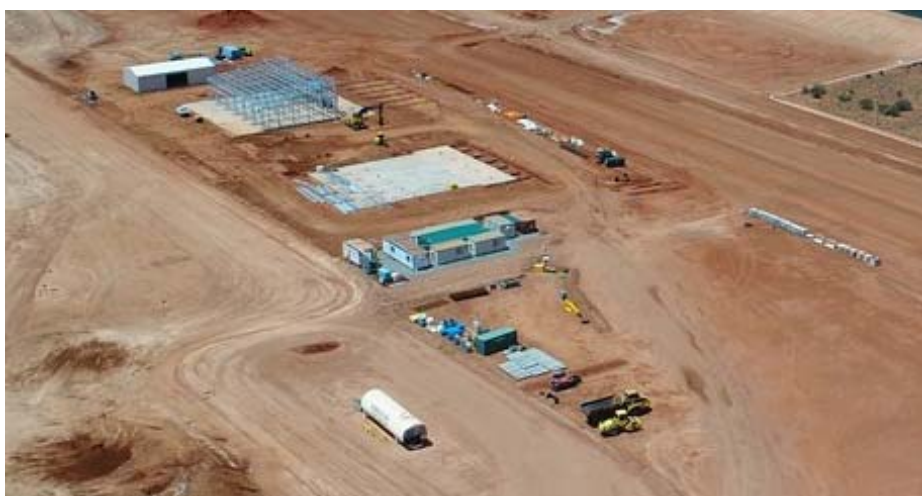
Gruyere 45 MW Powerhouse under Construction
